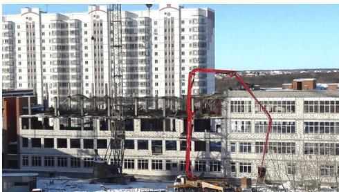
Figure 1: The Collapse of the floor slab during the construction of a school building in Kursk
